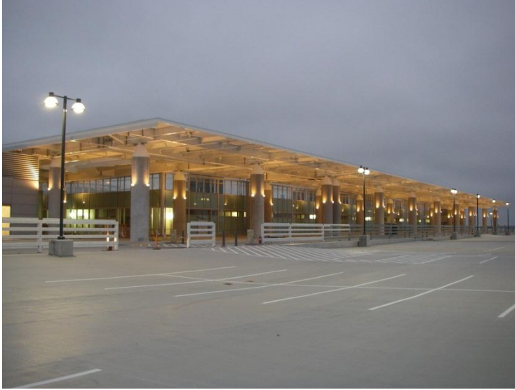
RCF Customer Service Building Lighting
