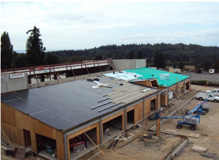
CNG Equipment Racks – Foreground BMF Building – Roofing & Sheathing Exterior
