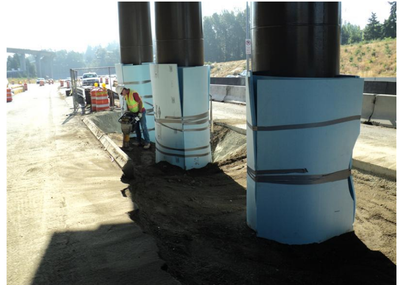
SR 99 Bridge Column Jackets and Backfill
